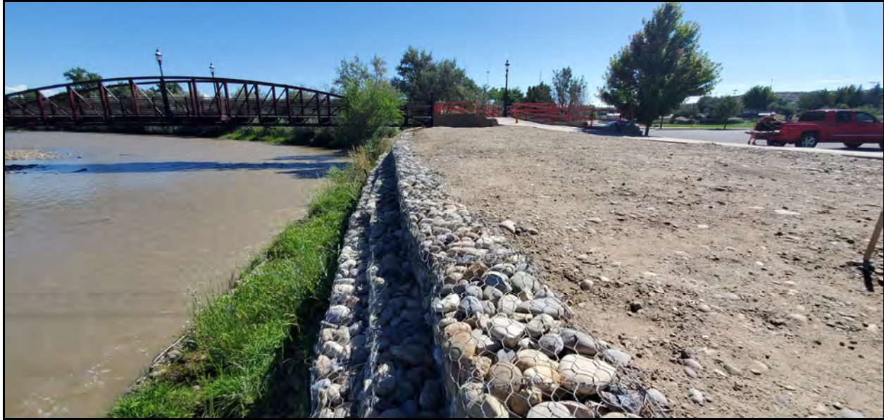
Existing Gabion Wall along Animas River near Boring B-5 View Towards the East
